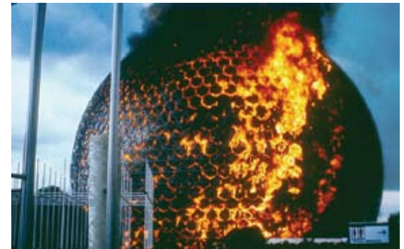
A fire in 1976 destroyed the acrylic shell of the Biosphere.
